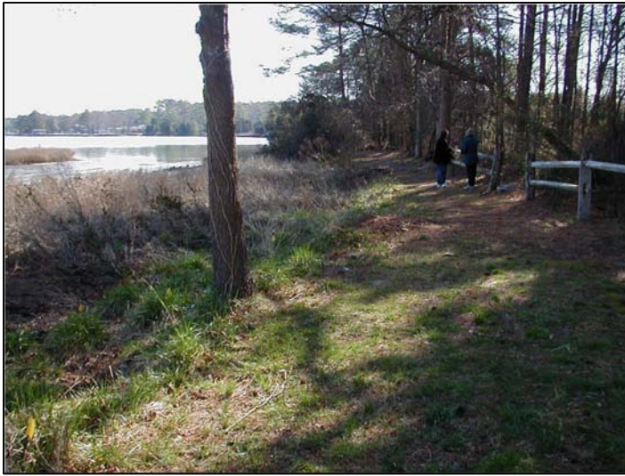
Bank erosion - low
