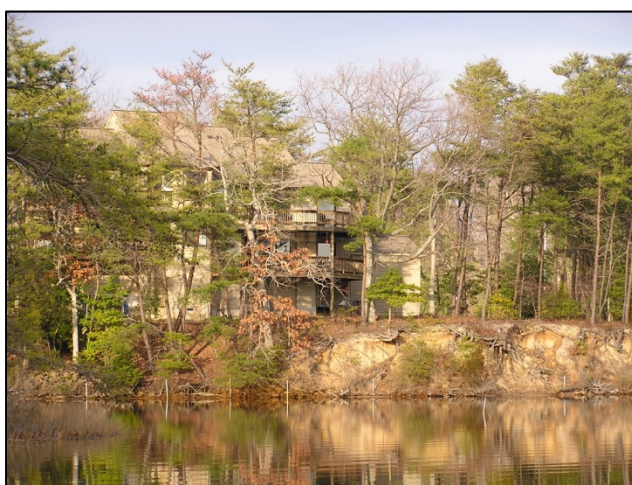
House too close to bank for grading back
