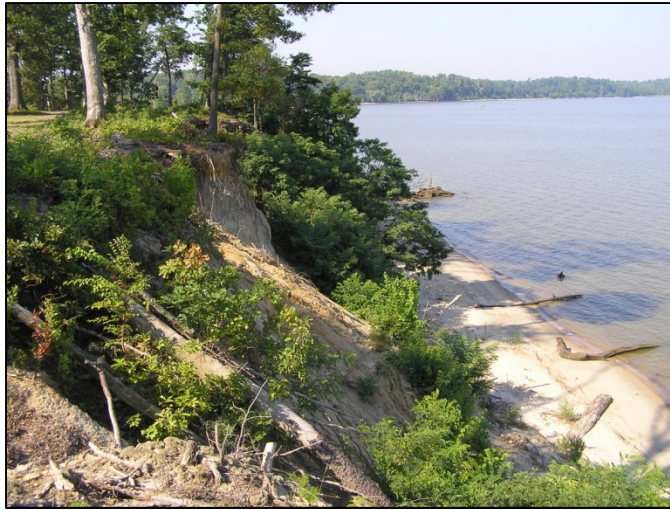
Bank erosion – high; forested shoreline; bank height > 30 ft
